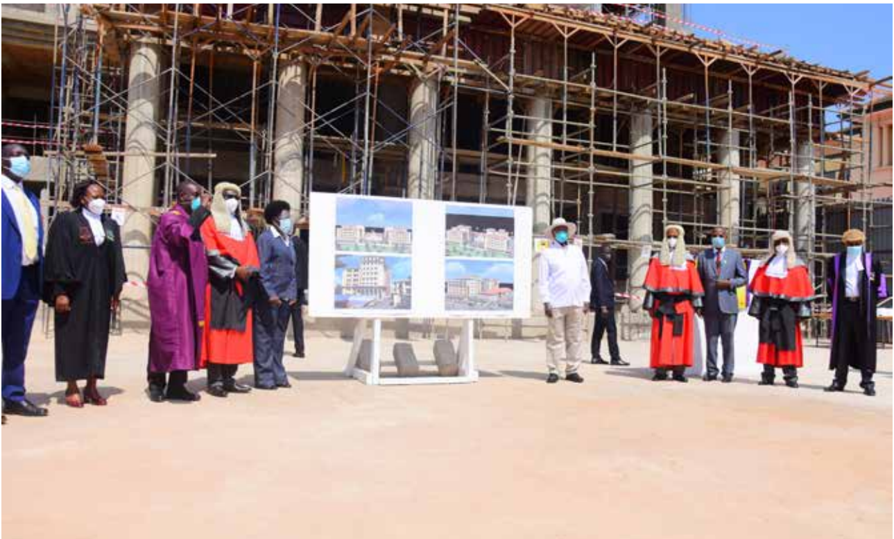
H.E. President Yoweri Kaguta Museveni laid the foundation stone for the Supreme Court and Court of Appeal buildings on February 5, 2021. This was during the Opening of the New Law Year event.
