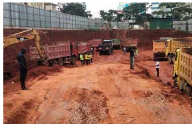
Earth works in March 2020.
